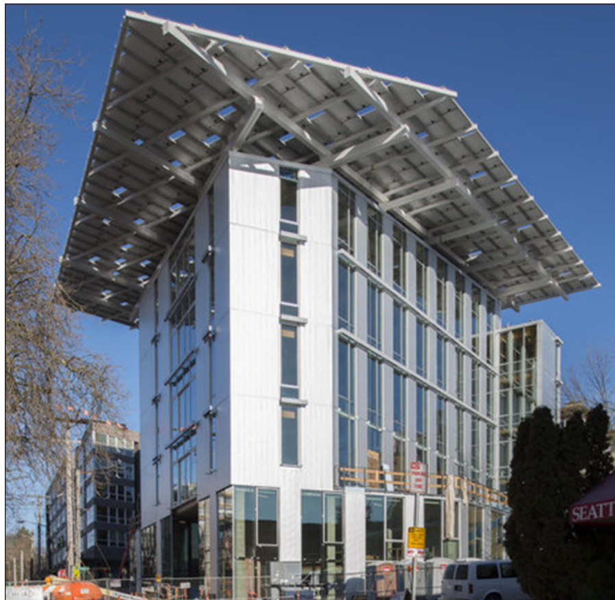
Figure 1—The Bullitt Center, Seattle, Washington. Some of the features of this building include net zero energy, net zero water, net zero carbon, composting toilets, toxic-free materials, and enhanced day lighting using high-performance windows. Even the shape of the roof appears to imitate a tree canopy.
